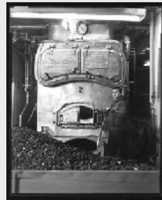
To bank a fire, fresh coal would be piled on top of the burning coals inside of the fire box. Piling the coal in this way reduced the amount of oxygen around the individual pieces, causing the fire to burn more slowly. If a fire was banked well, it would last until morning.
